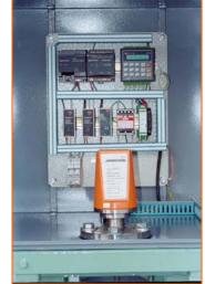
counterweight to prevent any part of the assembly making contact with the wall of the stilling tube. The pre-calibration status meant that once installed, the TDR unit was commissioned in a matter of
