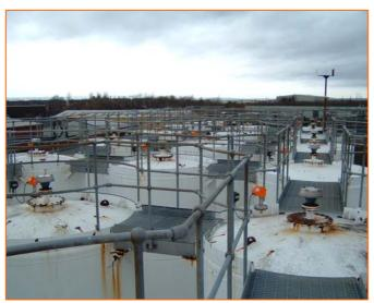
All the ATEX certified level measuring transmitters at the Caldic site are linked back via intrinsically safe barriers to a central control panel, which incorporates a versatile paperless chart recorder. This powerful instrument gives clear pictograms of the changing tank contents so that operators and management, either locally or
