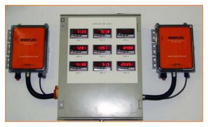
The Webflex system provides a number of key operational benefits and, because it runs on standard Internet Explorer, does not require any specialist software expensive or licenses. Each Webflex unit can take up to six 4-20 mA analogue inputs and six digital inputs. For Bendicks
